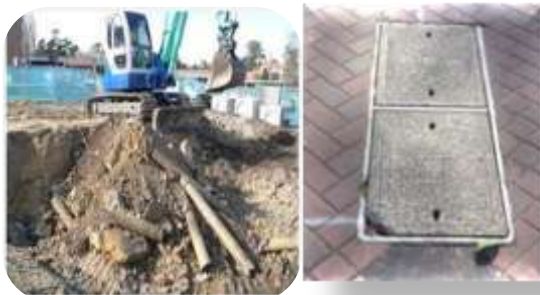
Pits & buried underground asbestos services
